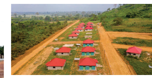
CONSTRUCTION OF STATE HOUSING PROJECT AT SEFWI WIAWSO
