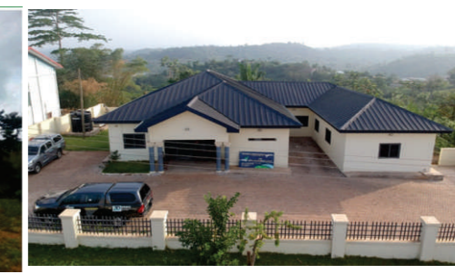
CONSTRUCTION OF DISTRICT HEALTH INSURANCE OFFICE
