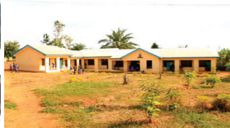
CONSTRUCTION OF 6-UNIT CLASSROOM BLOCK AT SEFWI ASAWINSO (GNPC)
