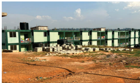
CONSTRUCTION OF 500 BED CAPACITY HOSTEL AT SEFWI WIAWSO NURSING TRAINING COLLEGE
