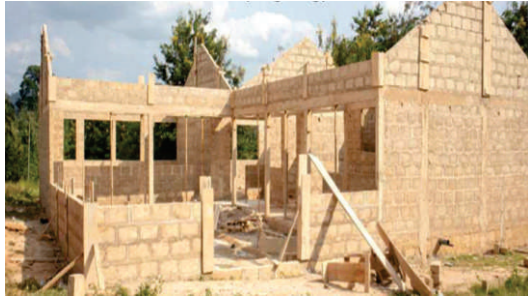
CONSTRUCTION OF KG BLOCK AT KUNUMA
