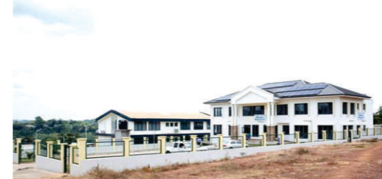
CONSTRUCTION OF BUSINESS RESOURCE CENTRE
