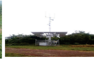
CONSTRUCTION OF COMMUNICATION MAST AT PARADISE
