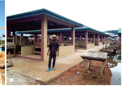
CONSTRUCTION OF 11No. 14-UNIT OPEN MARKET STALLS (MARKET COMPLEX)
