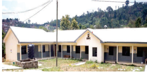
CONSTRUCTION OF 6UNIT CLASSROOM BLOCK AT SEFWI WIAWSO SEC TECH (GNPC)
