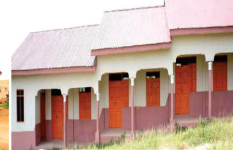
CONSTRUCTION OF 3UNIT CLASSROOM BLOCK AT SEFWI ABOBOYAA
