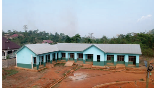
CONSTRUCTION OF CLASSROOM BLOCM AT ASAFO NURSING TRAINING
