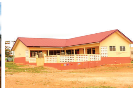
CONSTRUCTION OF KG BLOCK SEFWI BOSOMOISO
