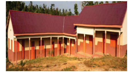
CONSTRUCTION OF 6UNIT CLASSROOM BLOCK AT ADEWANO
