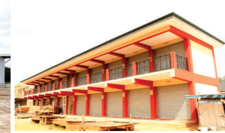
CONSTRUCTION OF 20 UNIT LOCKABLE STORES AT DWENASE MARKET
