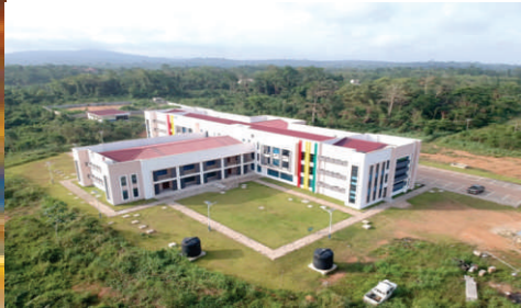
CONSTRUCTION OF REGIONAL COORDINATING COUNCIL
