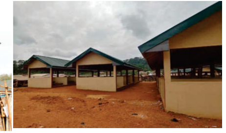
CONSTRUCTION OF STALLS AT DWENASE MARKET
