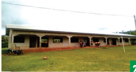
CONTINUATION OF 3UNIT CLASSROOM BLOCK AT PENAKROM
