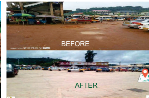
CONSTRUCTION OF FLOOR SLAP AT DWINASE STATION
