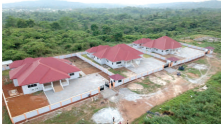
CONSTRUCTION OF SENIOR STAFF BANGALAW FOR RCC
