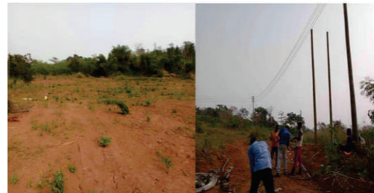
GRADING AND ELECTRIFICATION OF LIGHT INDUSTRIAL PARK
