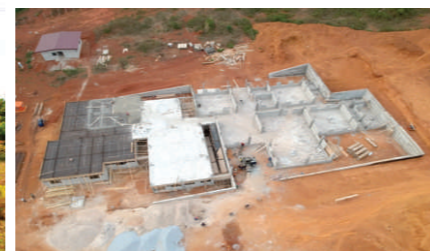
CONSTRUCTION OF TVET SCHOOL AT SEFWI BOAKO
