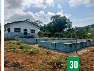
CONSTRUCTION OF HATCHERY POND AT SEFWI WIAWSO
