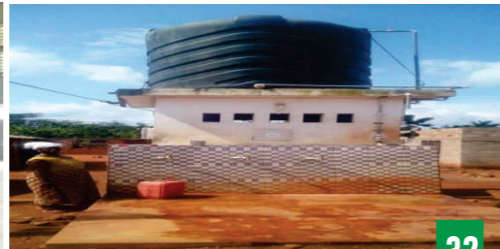
DRILLING AND MECHANIZATION OF BORE HOLE AT ASAWINSU MARKET AREA
