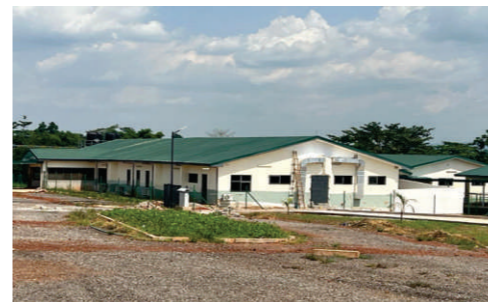
CONSTRUCTION OF INFECTIOUS TREATMENT CENTRE AT SEFWI ASAWINSO
