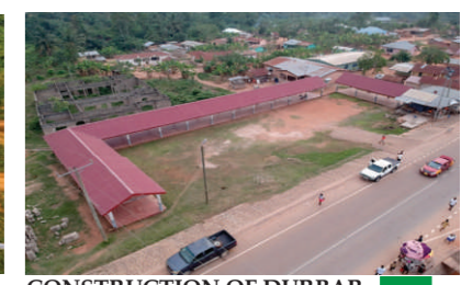
CONSTRUCTION OF DURBAR GROUND PUNIKROM
