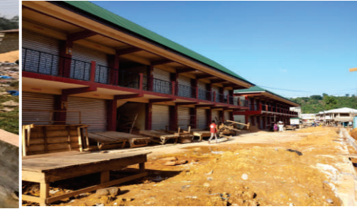
CONSTRUCTION OF 2No 2-STOREY 28 UNIT LOCKABLE STORES
