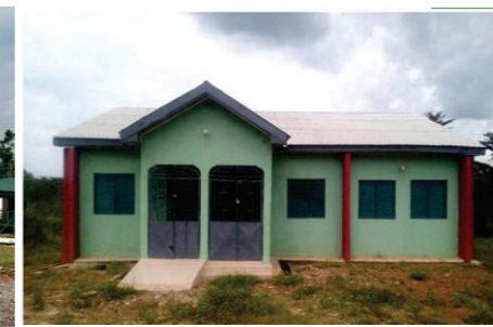
COMPLETION OF BOBRA CHPS COMPOUND
