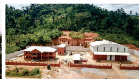
CONSTRUCTION OF ECG REGIONAL WAREHOUSE
