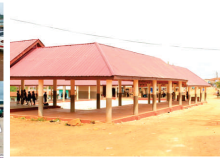
CONSTRUCTION OF DRUBAR GROUNDS AT AHWIAM
