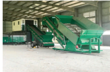
CONSTRUCTION OF WASTE TREATMENT PLANT AT ABOANIDUA
