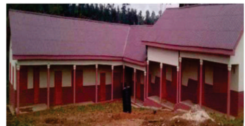
CONSTRUCTION OF 6UNIT CLASSROOM BLOCK AT AMPABAME
